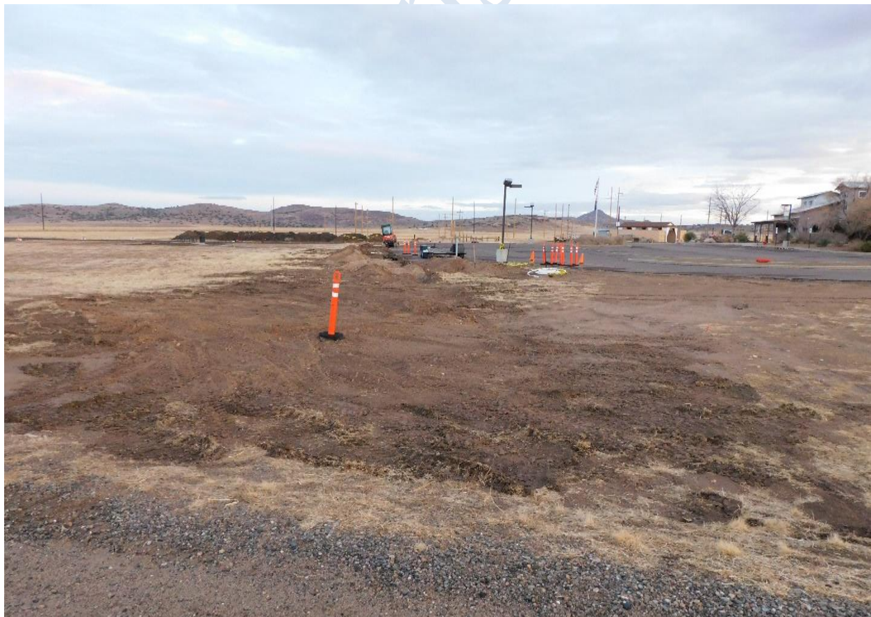
Burying of new electrical service
