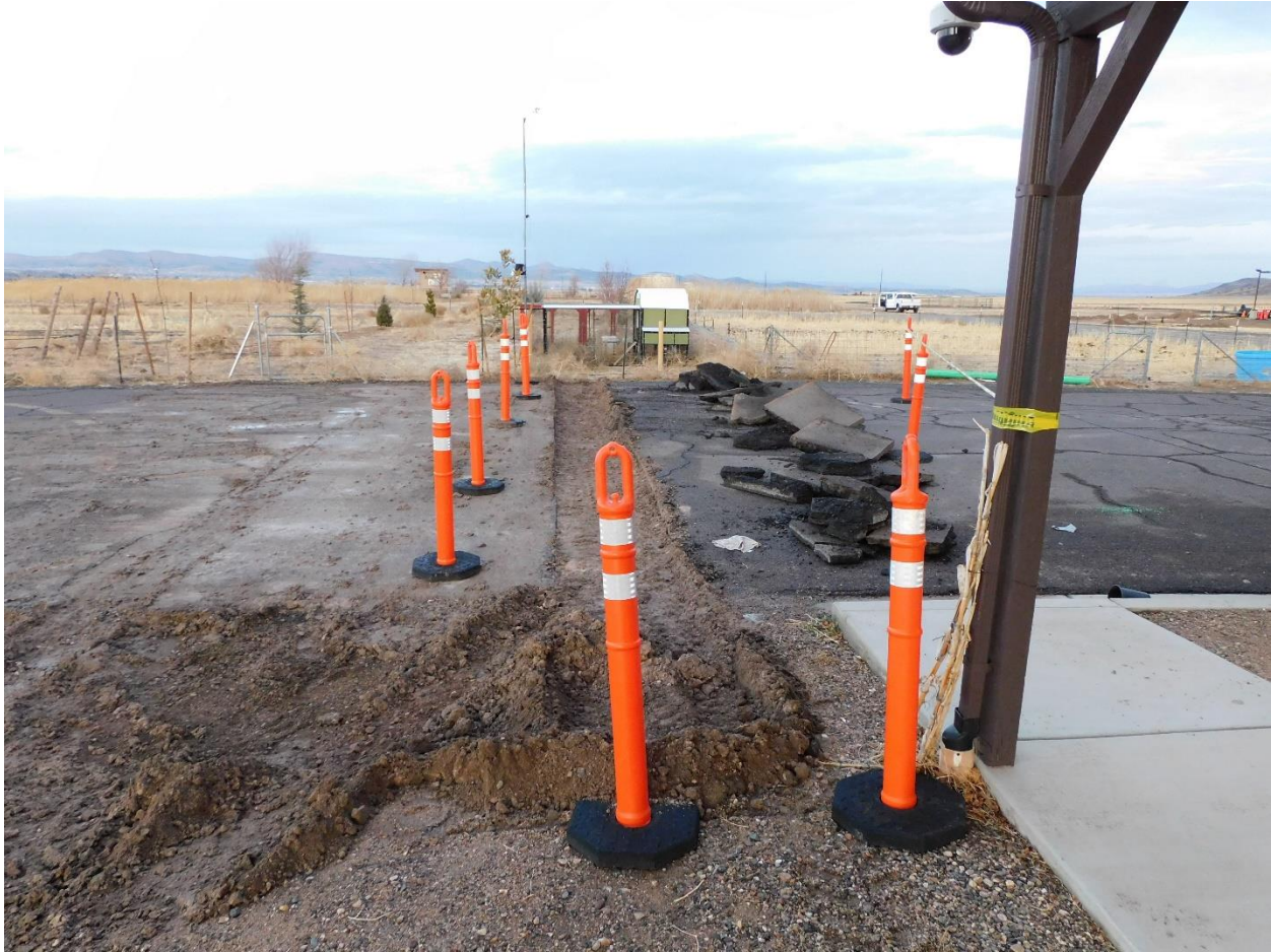
Bringing electrical service from Building 55
