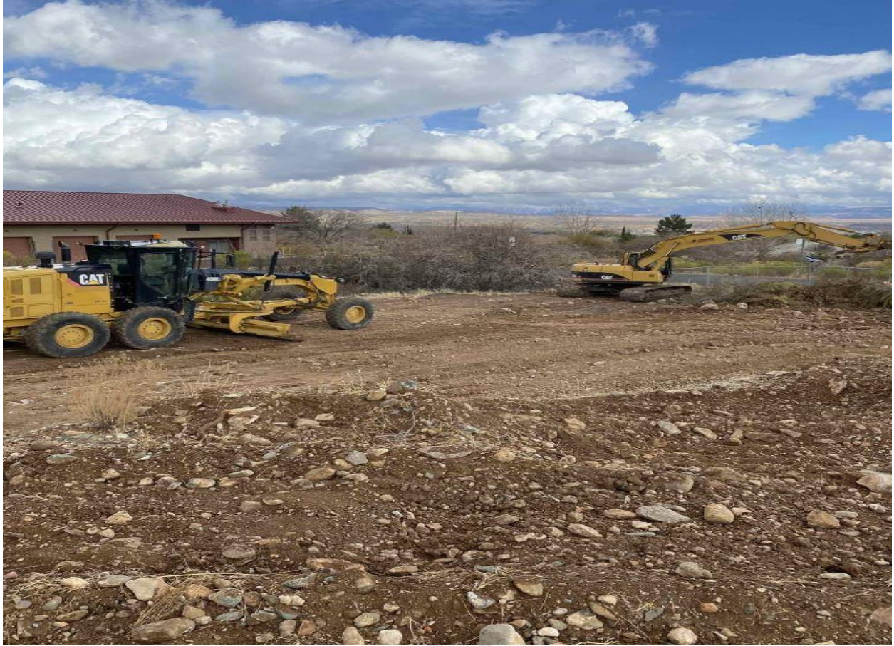
Excavation begins for building pad and utilities
