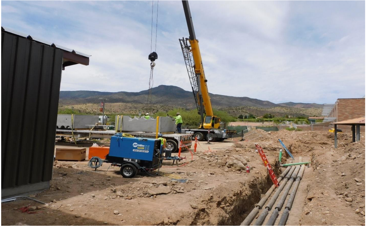
Craning utility vaults – 21,500 and 16,000 pounds
