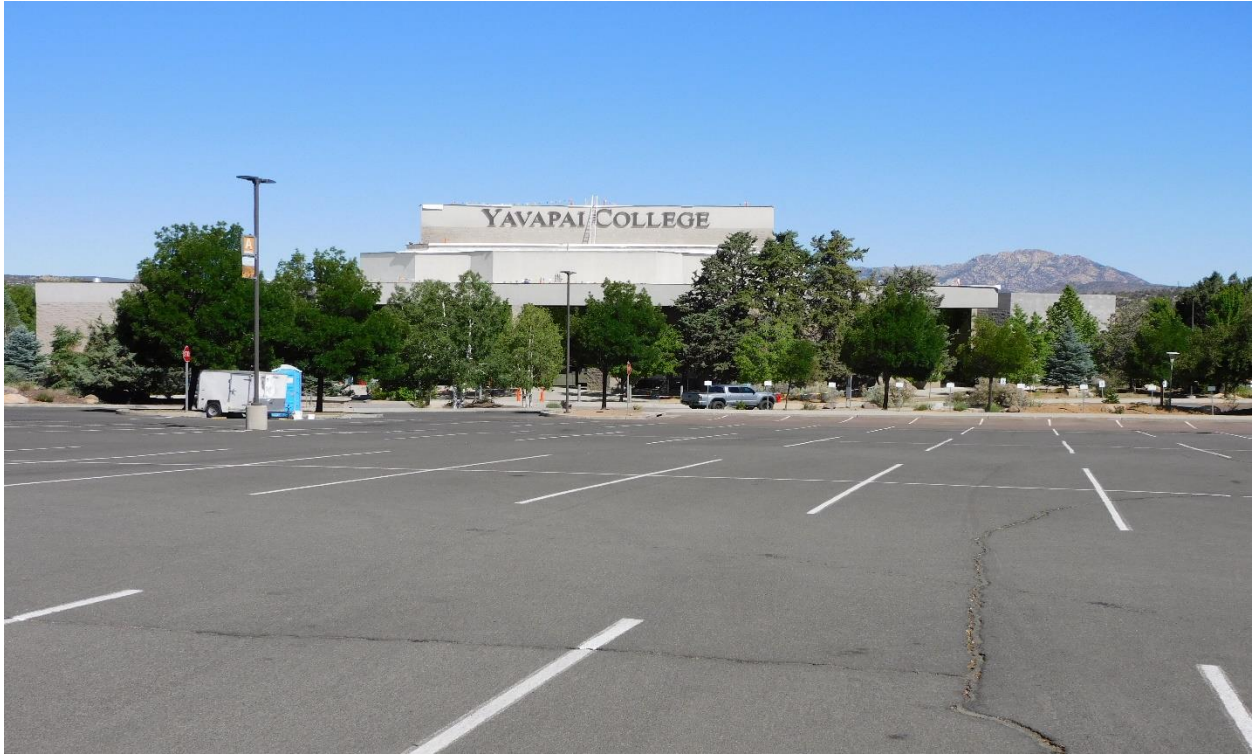
PAC roof replacement
