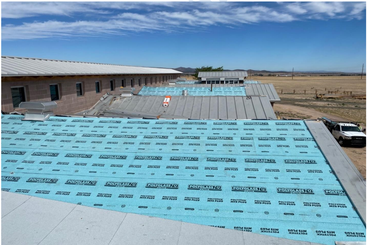
Chino Valley Agribusiness Center roof replacement
