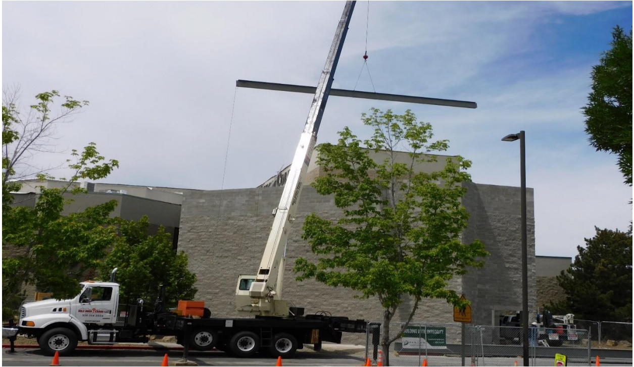
Craning beams for the roof structure
