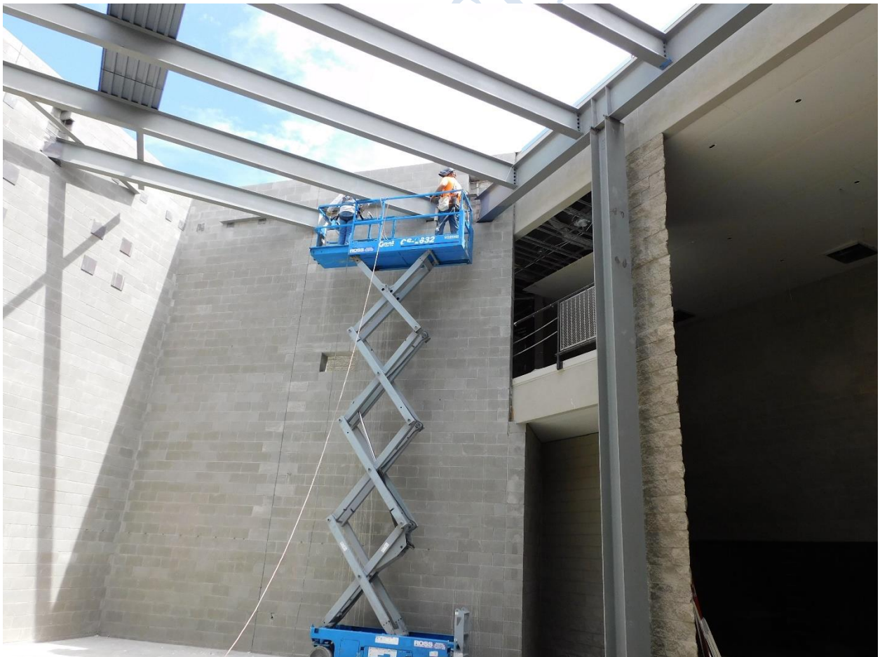
Welding beams for the new roof
