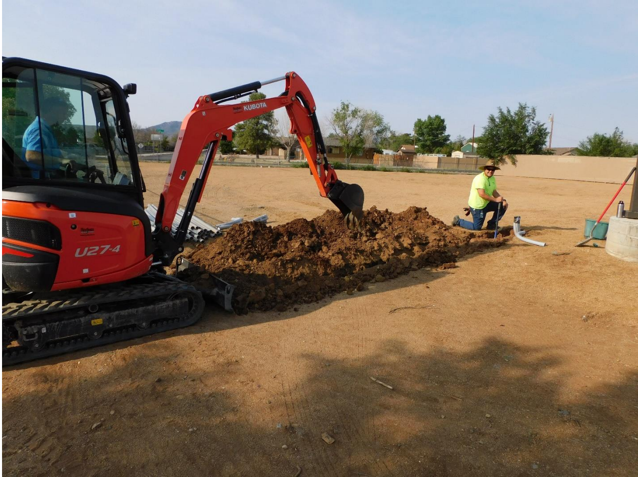
Brandon Biro and James Crockett installing electrical services for new marquee
