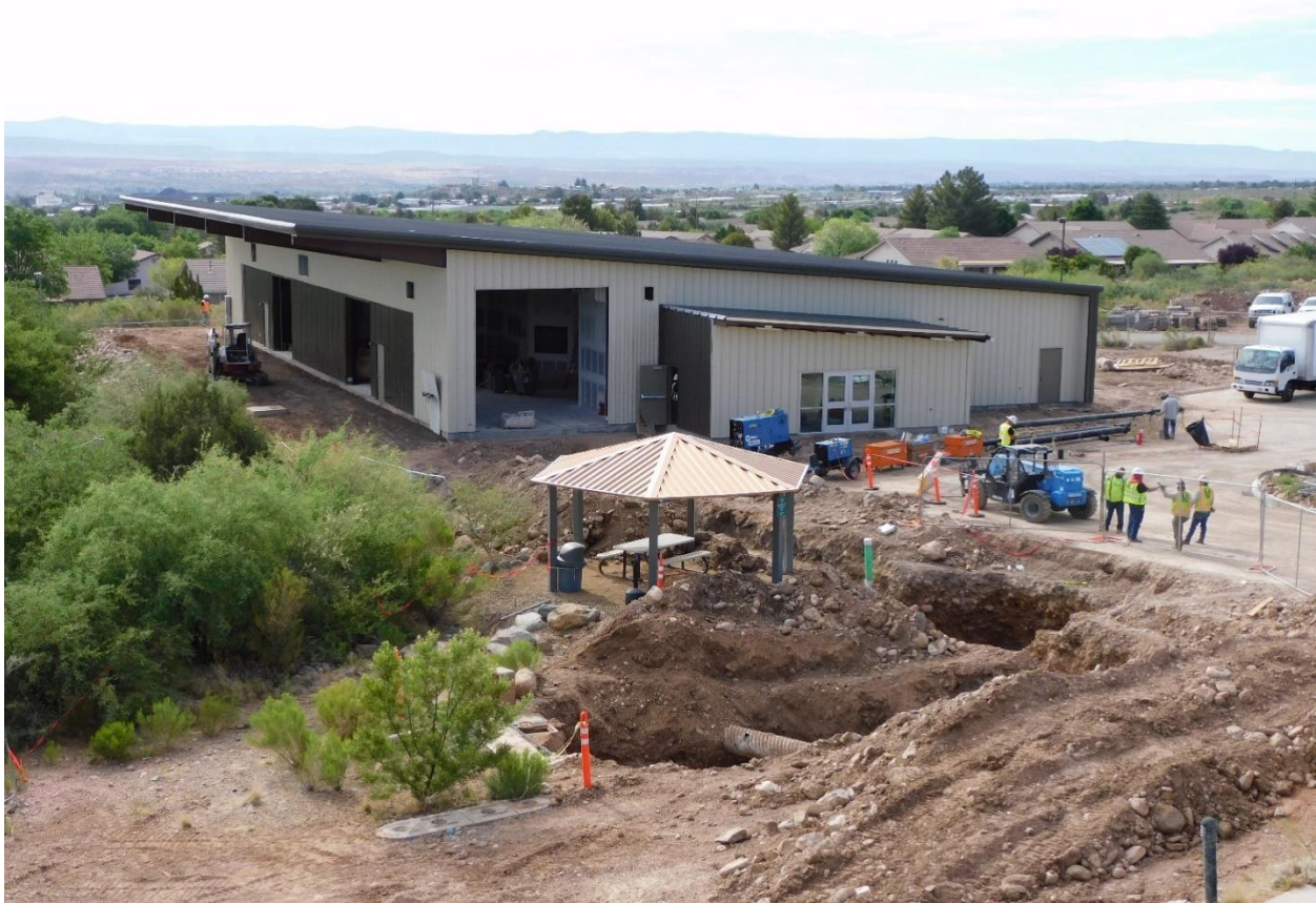
Trenching for utility placement
