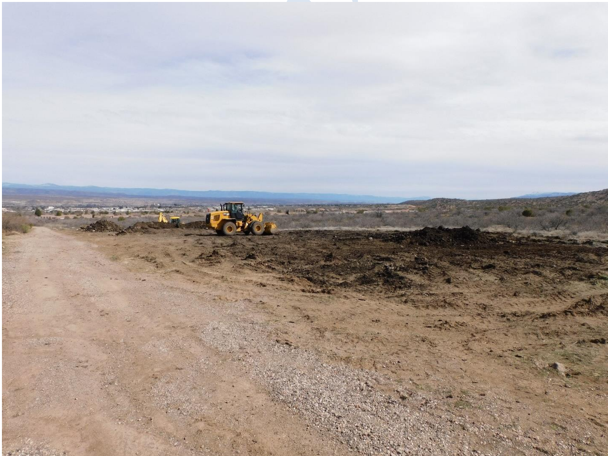
RV park construction activity east of upper vineyard
