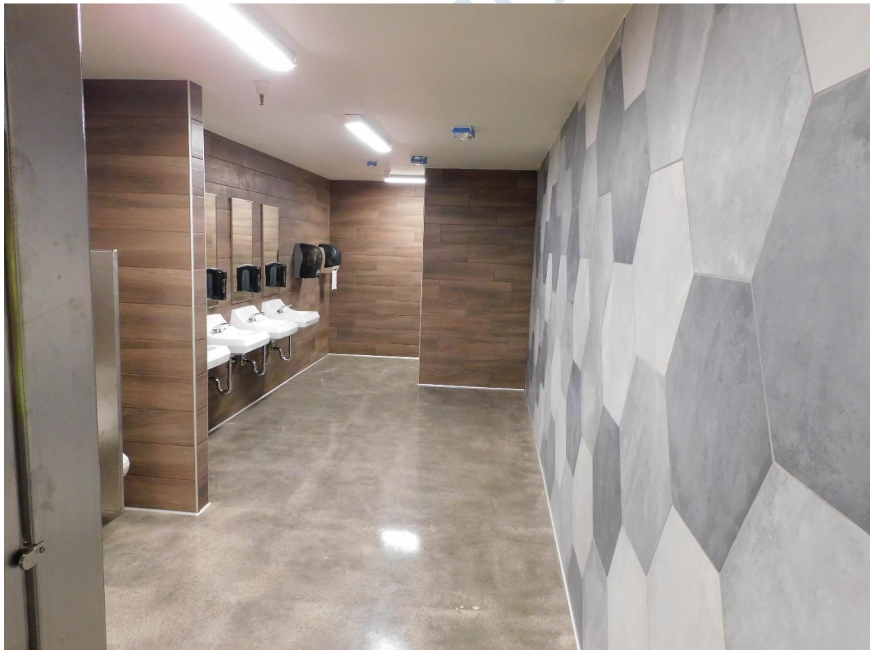
North restroom renovations at CTEC
