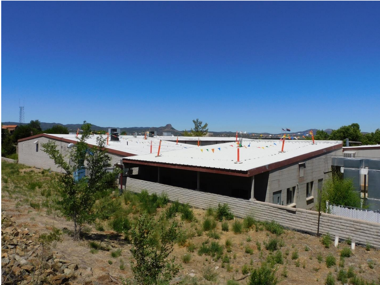
Roof repair and rooftop unit replacement Building 7
