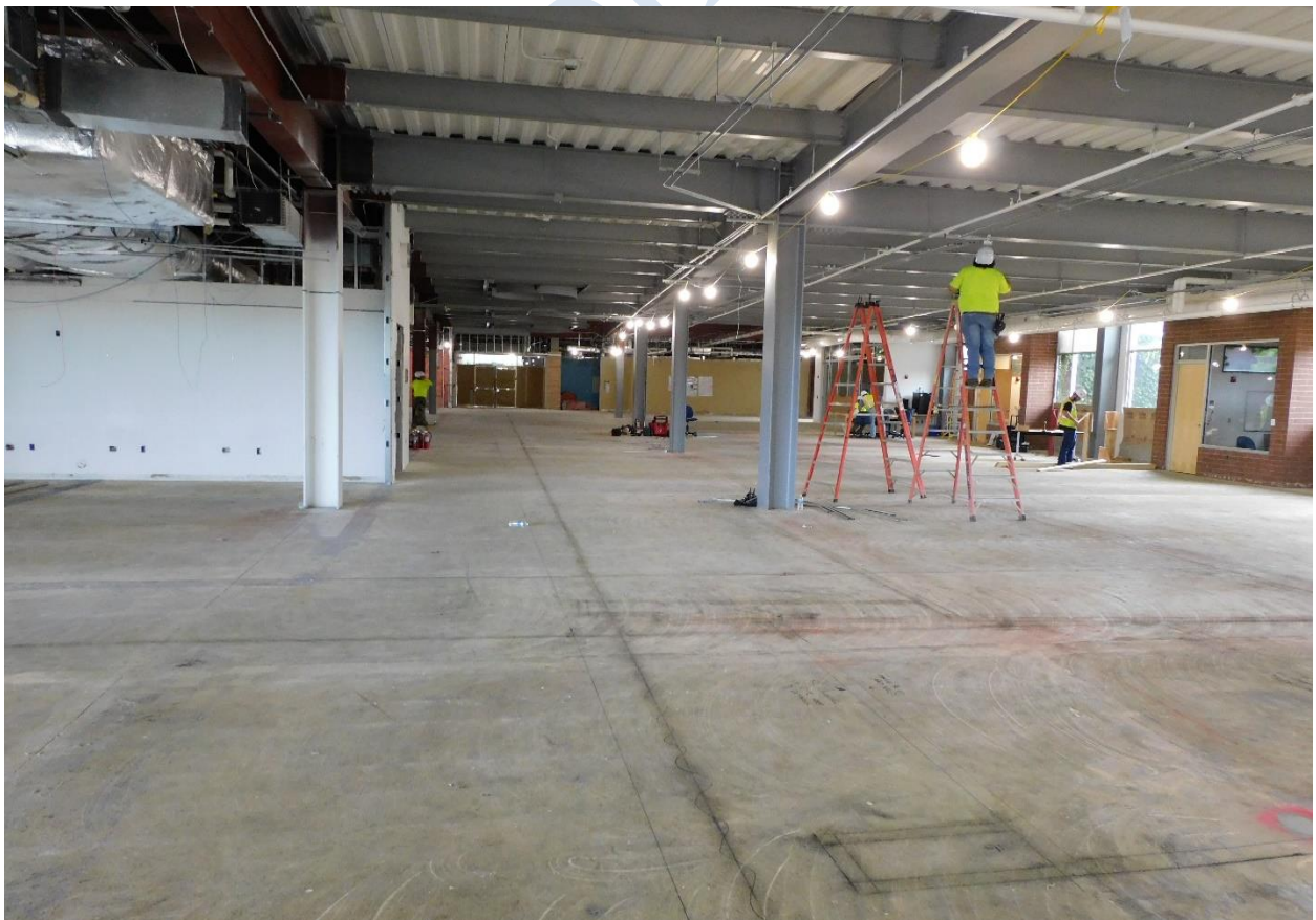
Layout for future metal studs to construct new walls
