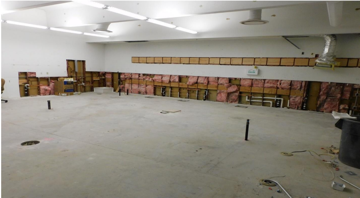
Culinary Building 4 room 220
