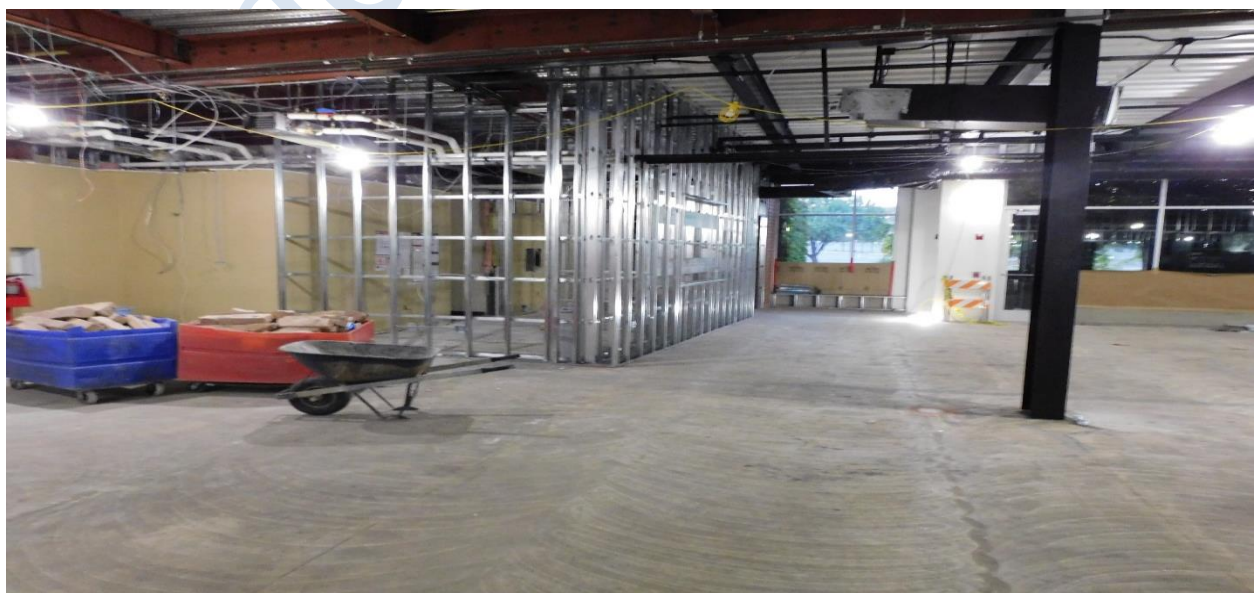
Framing new Yavapai College Foundation offices on the first floor
