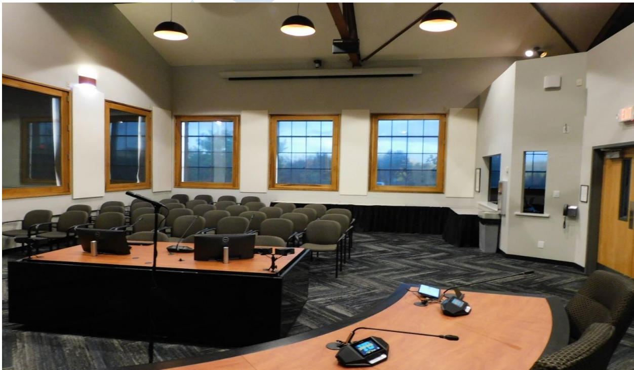
New acoustical wall and ceiling panels and window for tech booth
