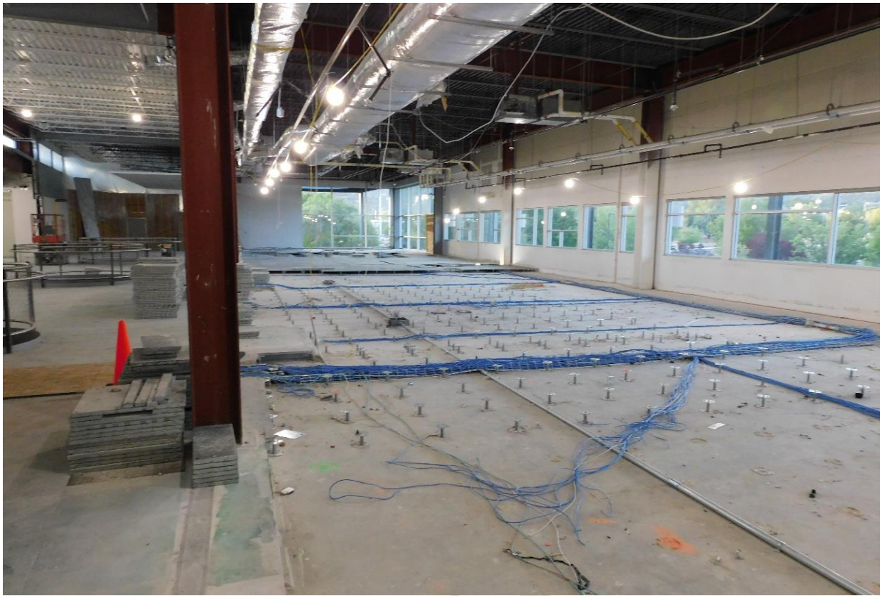
Second-floor computer commons looking south
