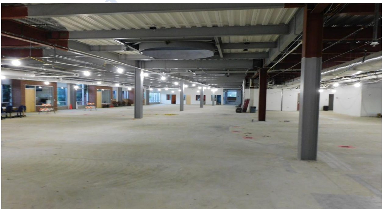
Library in Building 19
