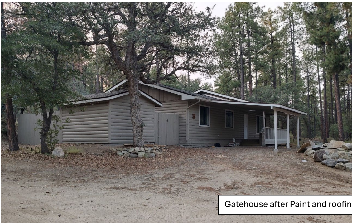
Gatehouse exterior ready for roofing and paint/stain
